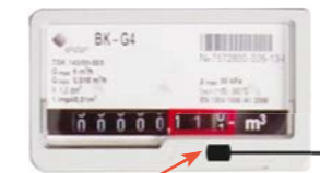
Built-in magnet in the gas meter
